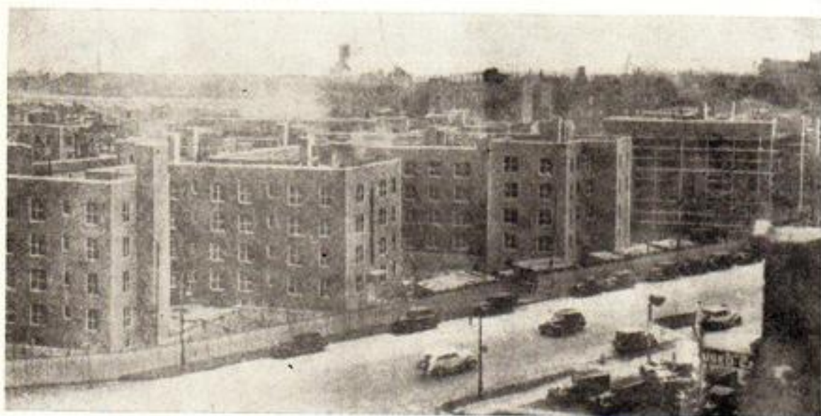
The PWA workers who put up these apartments at 153rd Street and the Harlem river, designed for low income groups to solve New York City's housing problem, will not live in them—for prospective tenants must show a bank account and have a job.
